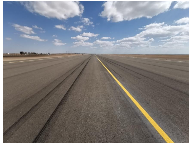
Breaking marks on TWY-A
